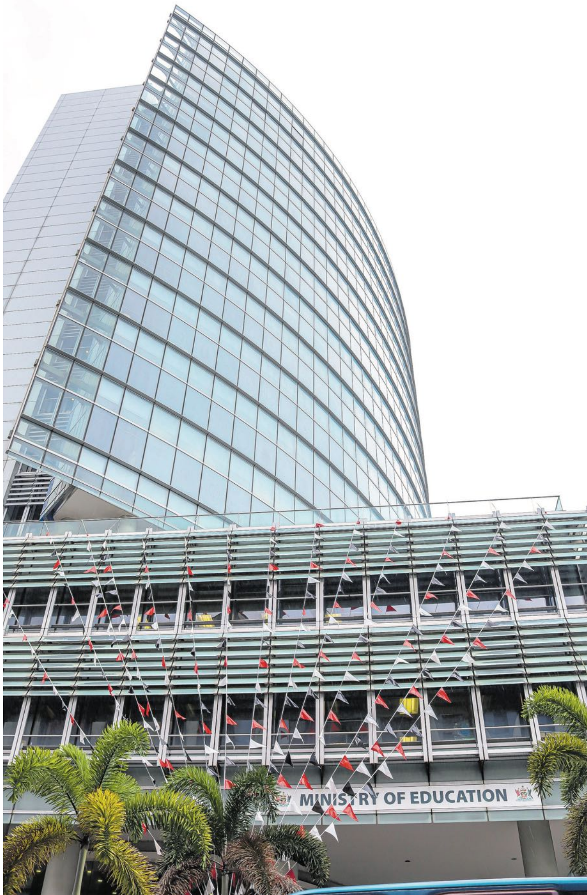
The Ministry of Education, St Vincent Street, Port of Spain.
