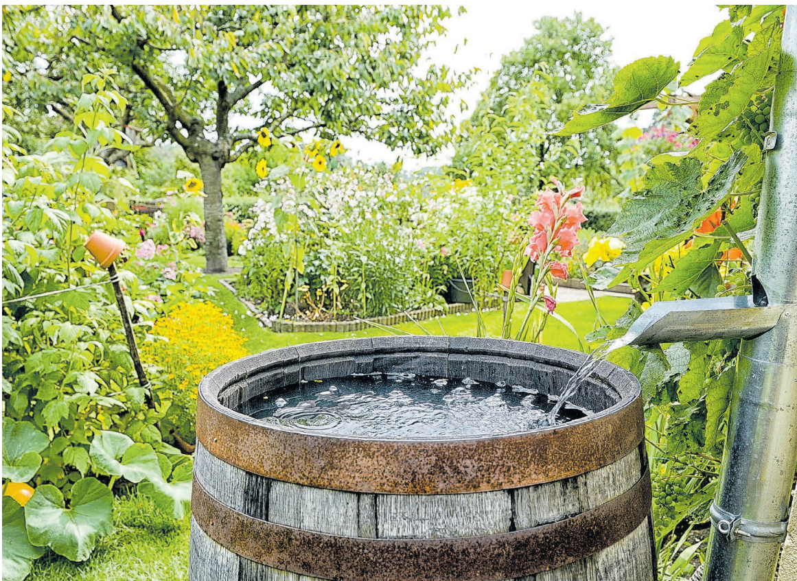
Rainwater harvesting. SOURCE: YGRENE.COM
