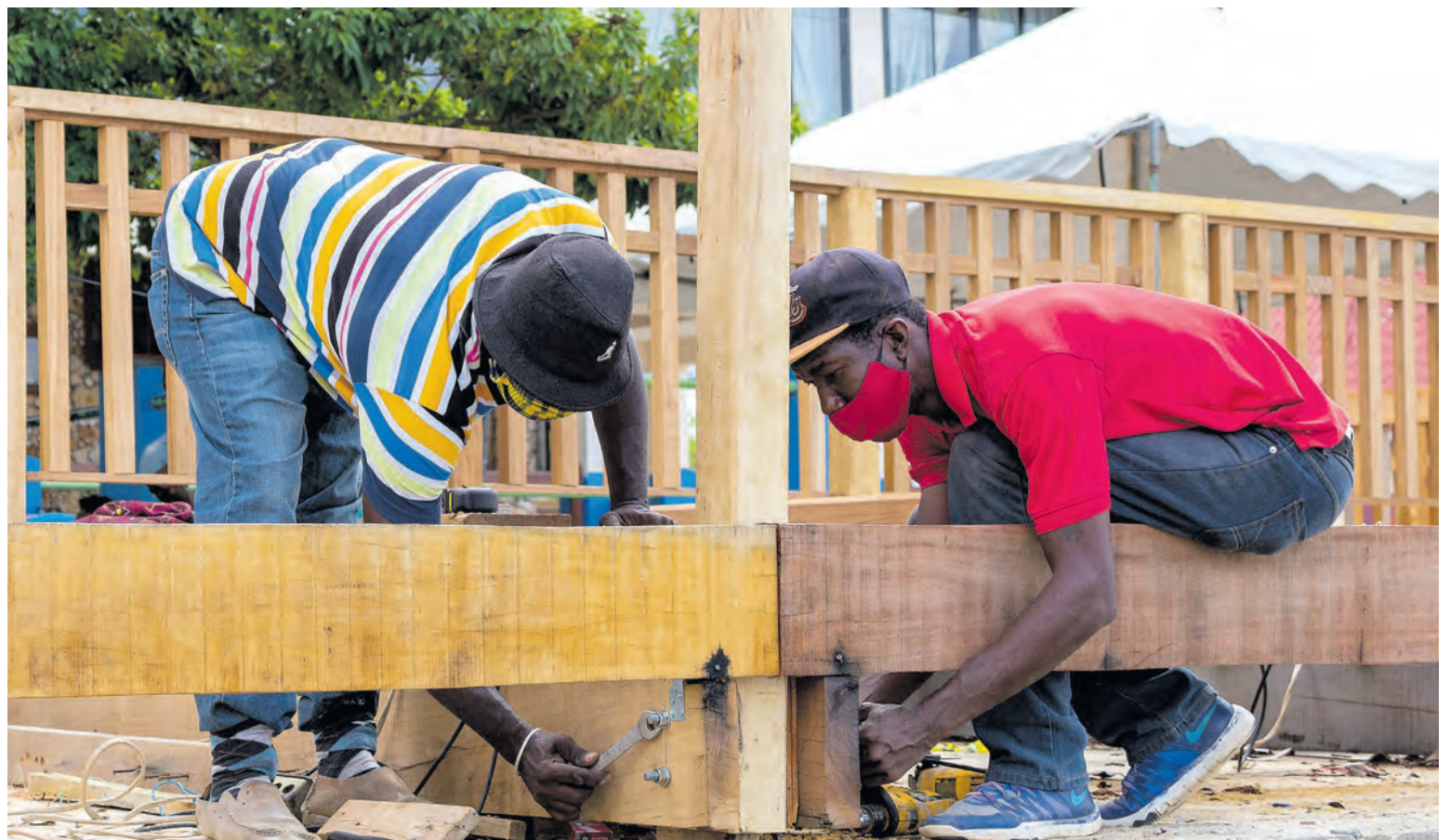
Workmen at the Buccoo Bay boardwalk site.
