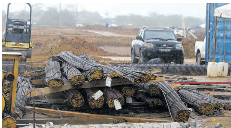
Steel rods at the Phoenix Park Industrial Estate construction site.
