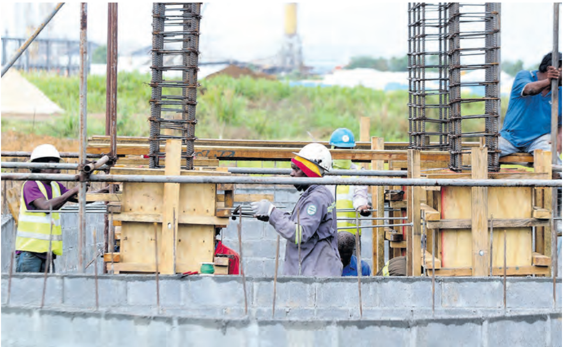
Construction at Phoenix Park Industrial Estate. PHOTO BY ANGELO MARCELLE
