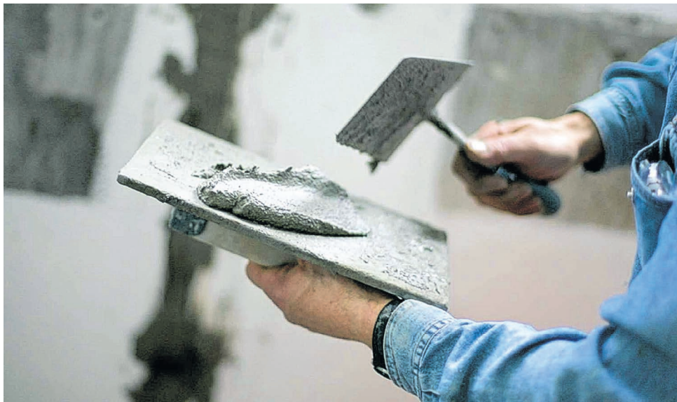
Make sure the plaster has dried completely before painting. PHOTO TAKEN FROM BNBARCHITECTS.BLOGSPOT.COM
